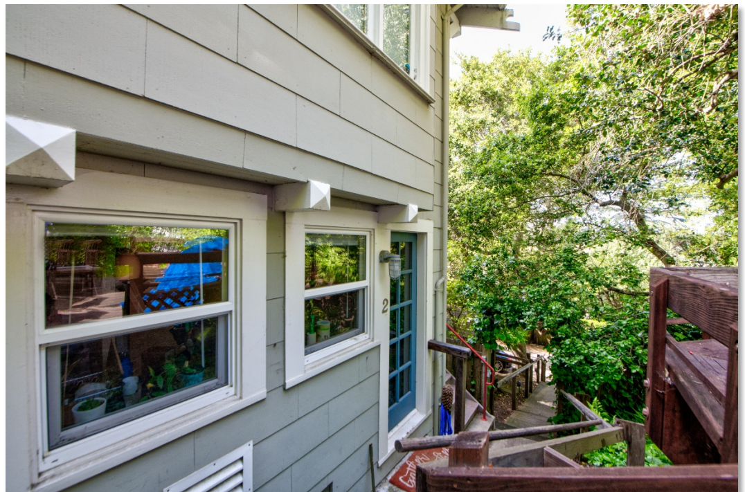
Entry to Apartment 2
