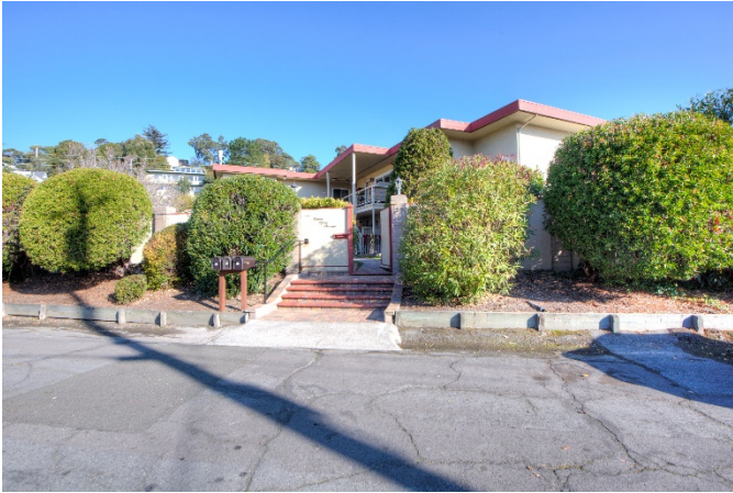
COMPLEX ENTRY FROM MOORING ROAD
