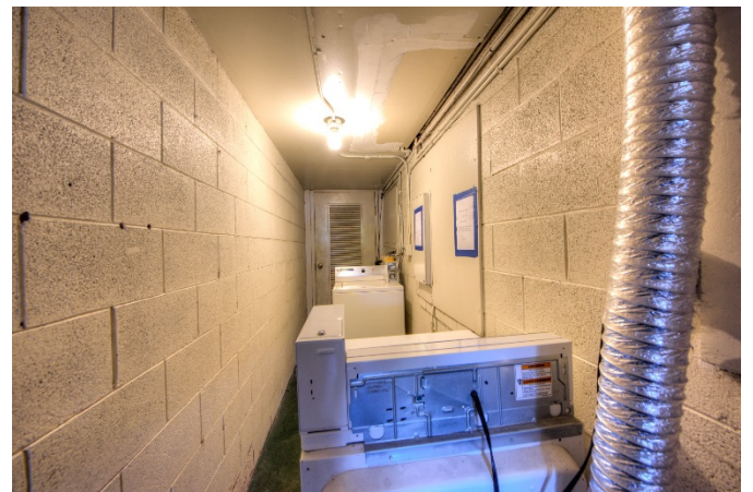
COMMON LAUNDRY ROOM
